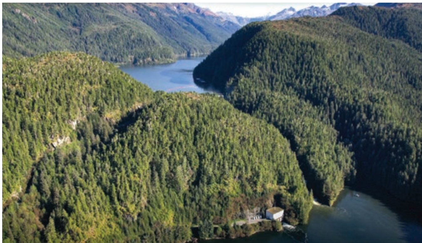
The Green Lake Hydro Project. Photo by Lee House.
